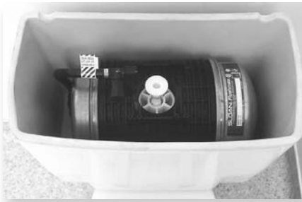
FLUSHMATE uses pressure-assist technology.
